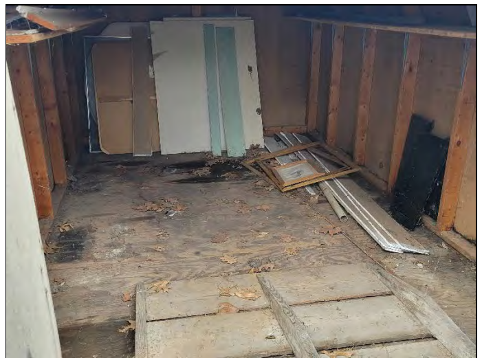
18. Subject – Interior of the shed
