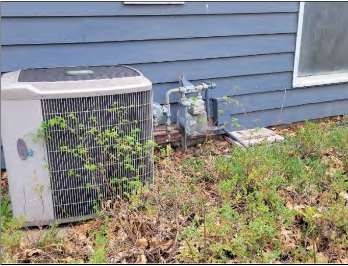
13. Subject – A/C unit and gas connection
