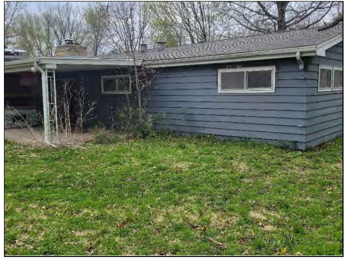
8. Subject (from the southwest corner)
