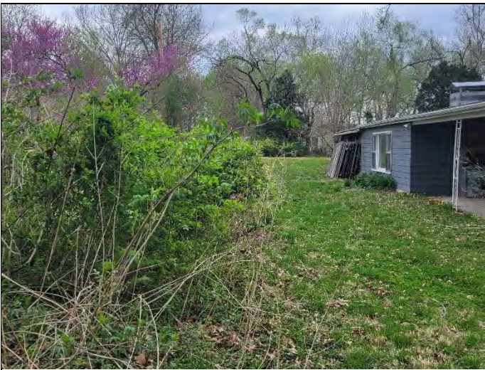
9. West portion of the Subject (from the southwest corner)
