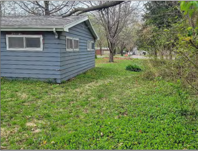
7. South portion of the Subject (from the southwest corner)
