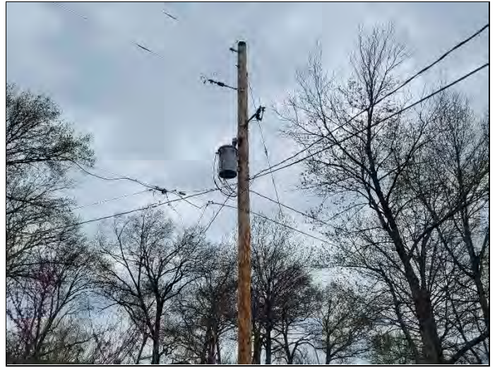
14. Subject boundary – Pole-mounted transformer
